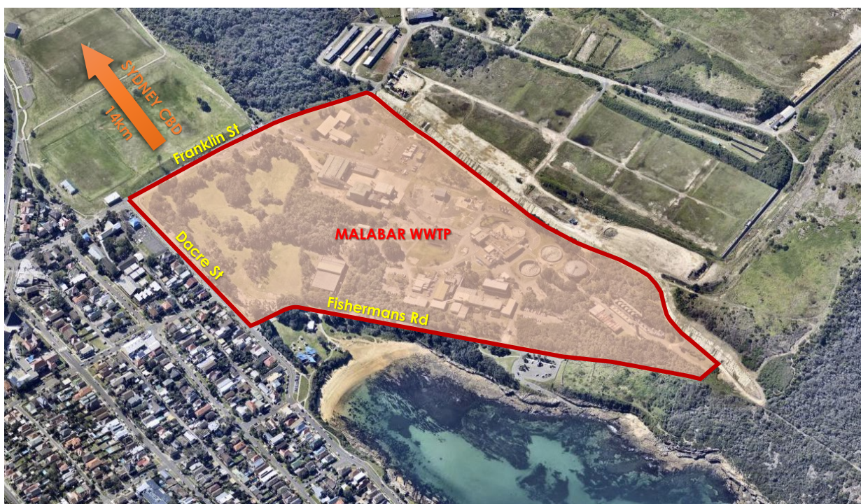
Figure 29: Malabar Wastewater Treatment Plant (Source: Nearmap)
